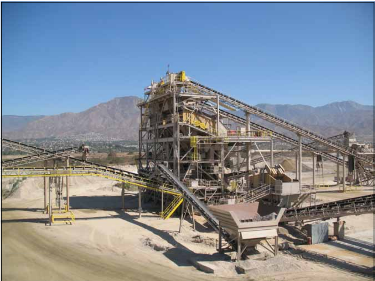
Cemex's Orange Street Plant, Highland, Ca.
